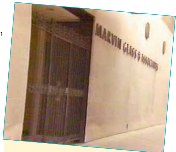
ABOVE The front entrance of the studio with the iron gate acting as the first line of security.
